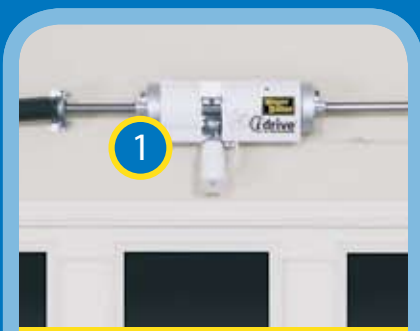
idrive mounts to the counterbalance above door.
