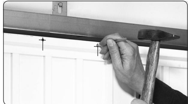
2. Punch in the fixing holes in the door frame with the aid of the enclosed spike.
