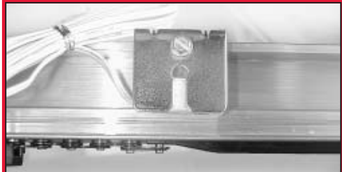
FIG. 7-2 Place “Open” limit switch.
