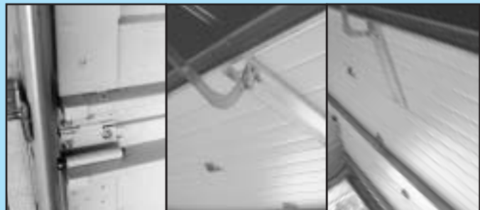
FIG. 2-6 Examples of door bracing.
