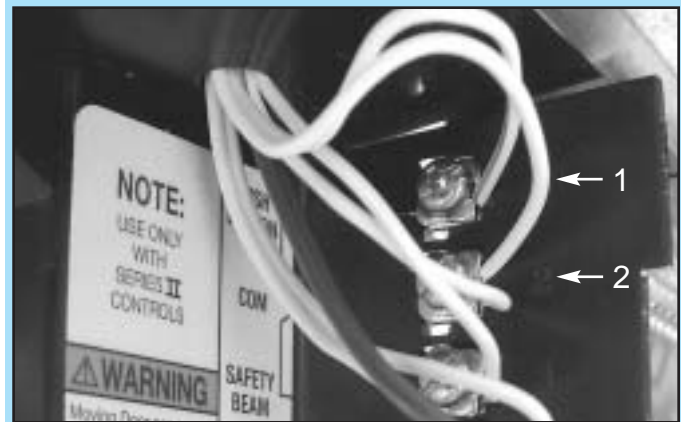
FIG. 5-1 Terminal attachments at power head.
