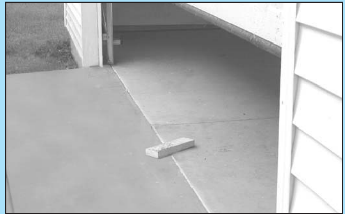
FIG. 6-6 2 x 4 under center of door opening.
