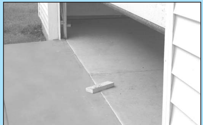
FIG. 6-5 2 x 4 under center of door opening.
